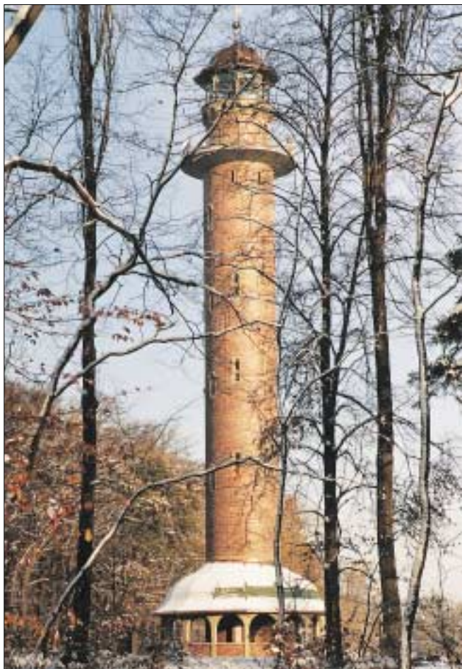
A fire observation tower at the Forest and Nature Education Centre in Jezioro Wysokie
